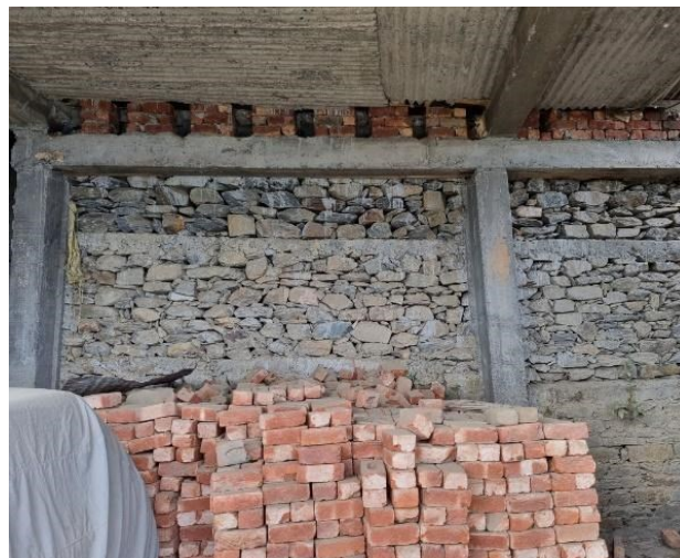
Fig. 10: Stone wall with RCC columns, slabs and concrete band Source: Author, 2022
