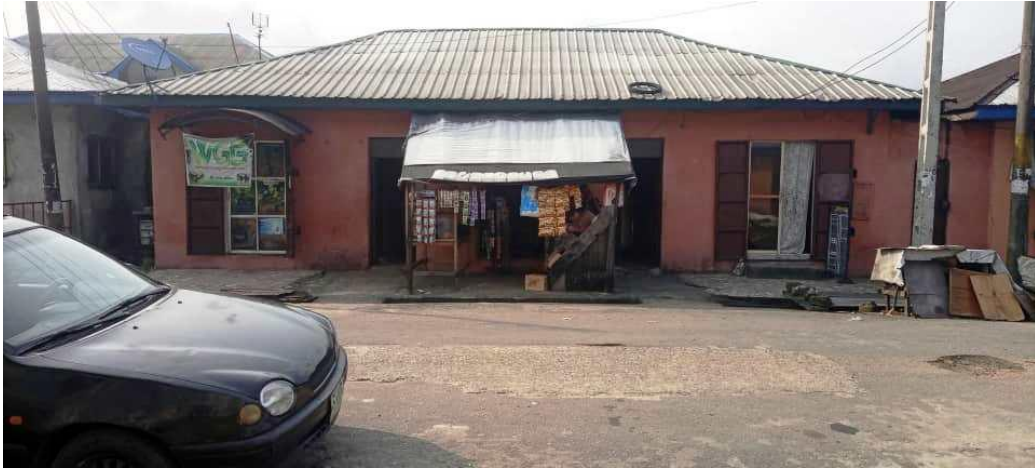
Fig. 5: Approach elevation of typical bungalow in Diobu (the canopy in the front with a shop is an unauthorized addition)
