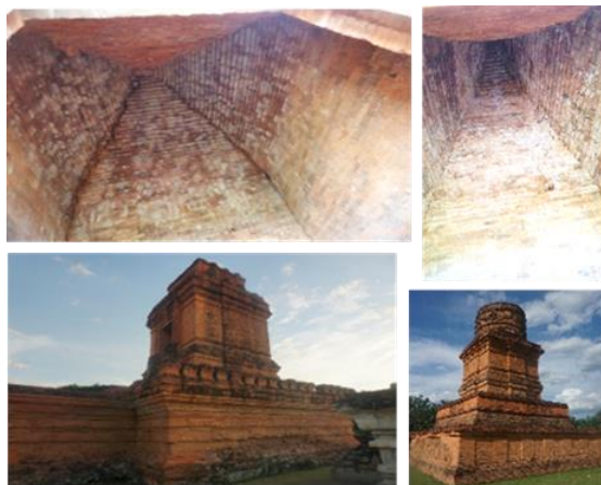
Fig. 10: Brick Temple in North Sumatra using the terraced corbel such as Si Pamutung and Bahal Temple Source: Herwindo, 2022
